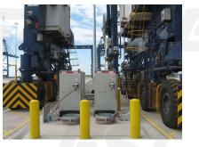
Daisy-chaining several MV Disconnect Cabinets minimizes the number of MV circuit breakers needed at the switchgear reducing the space required & electrical equipment cost.
